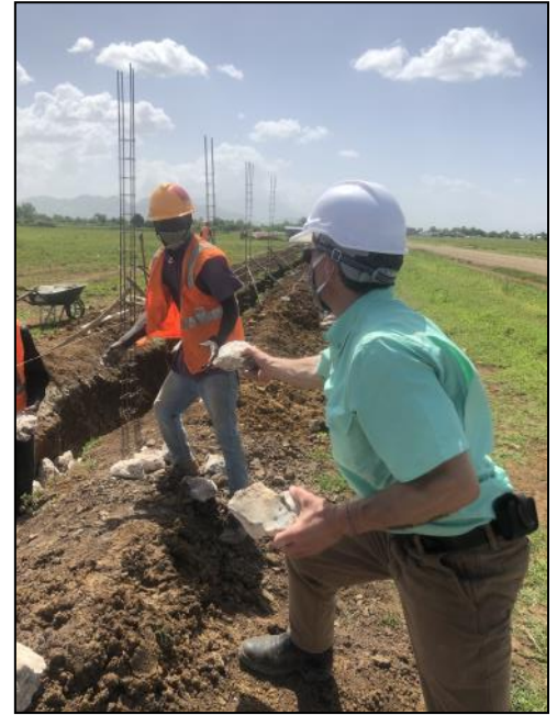
THP Director of New School Construction Jimi Grondin assists in placing the first stones in the foundation of the perimeter wall of LCS 2.
