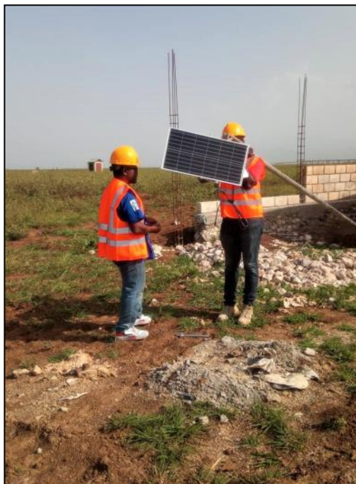
Above: Workers install solar-powered lights to illuminate the grounds at the building site. Above right: Workers construct the front perimeter wall of LCS 2. Right: Patrick Brun, head of THP's partner foundations in Haiti and Haitian private-sector leader (kneeling, center), with workers laying stones for the foundation of the perimeter wall of LCS 2.
